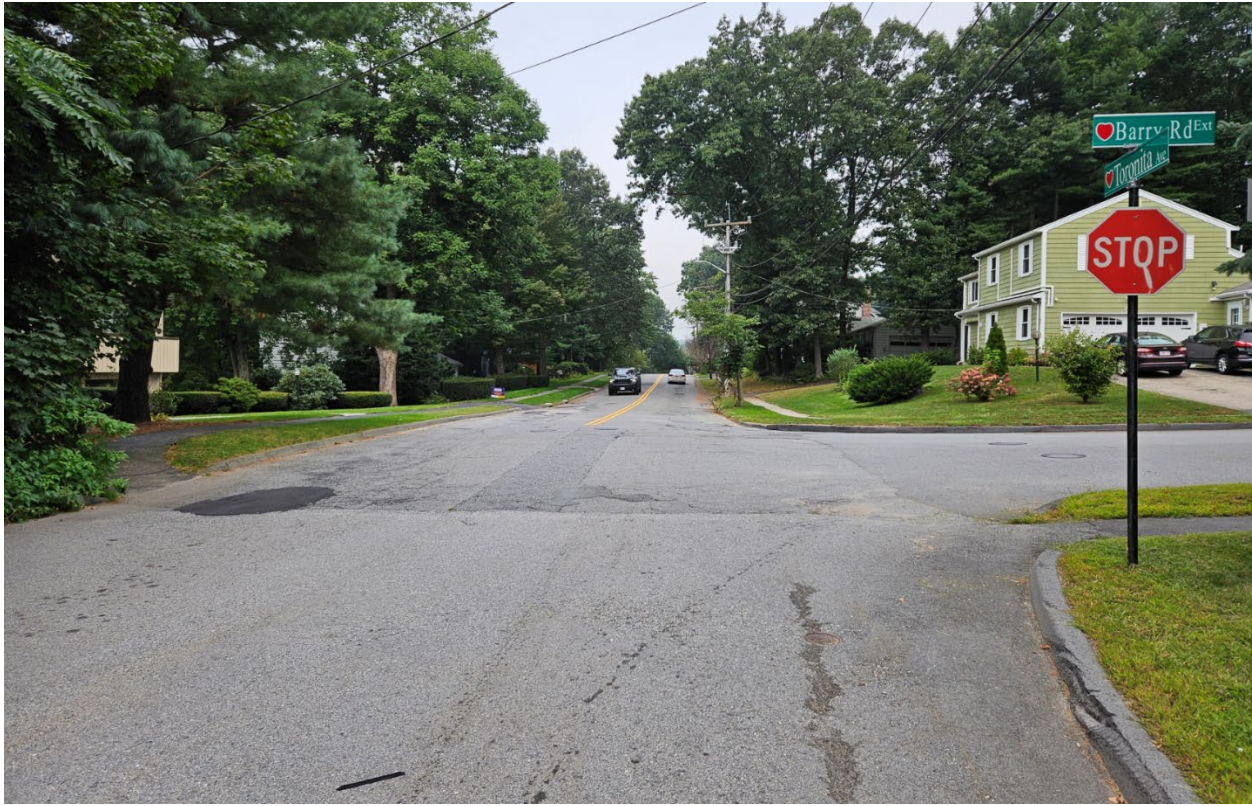
Figure 3: View westbound on Toronita Ave approaching Barry Rd and Barry Rd Ext (source: 9/8/2023 DTM site visit)
